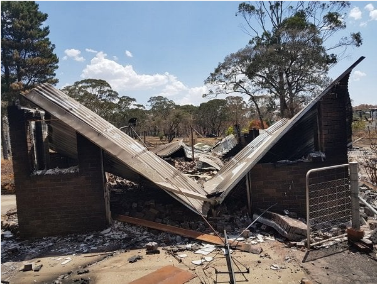
The gutted building of Sri Om center. Raining embers picked by furious winds gutted the building in no time.
